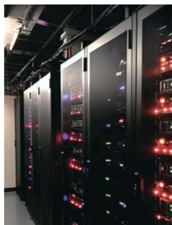
Uninterruptible Power Supply
