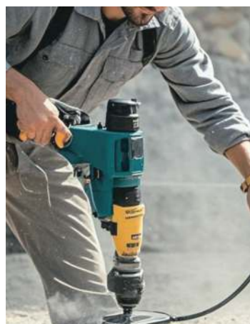
Outdoor Construction Work
